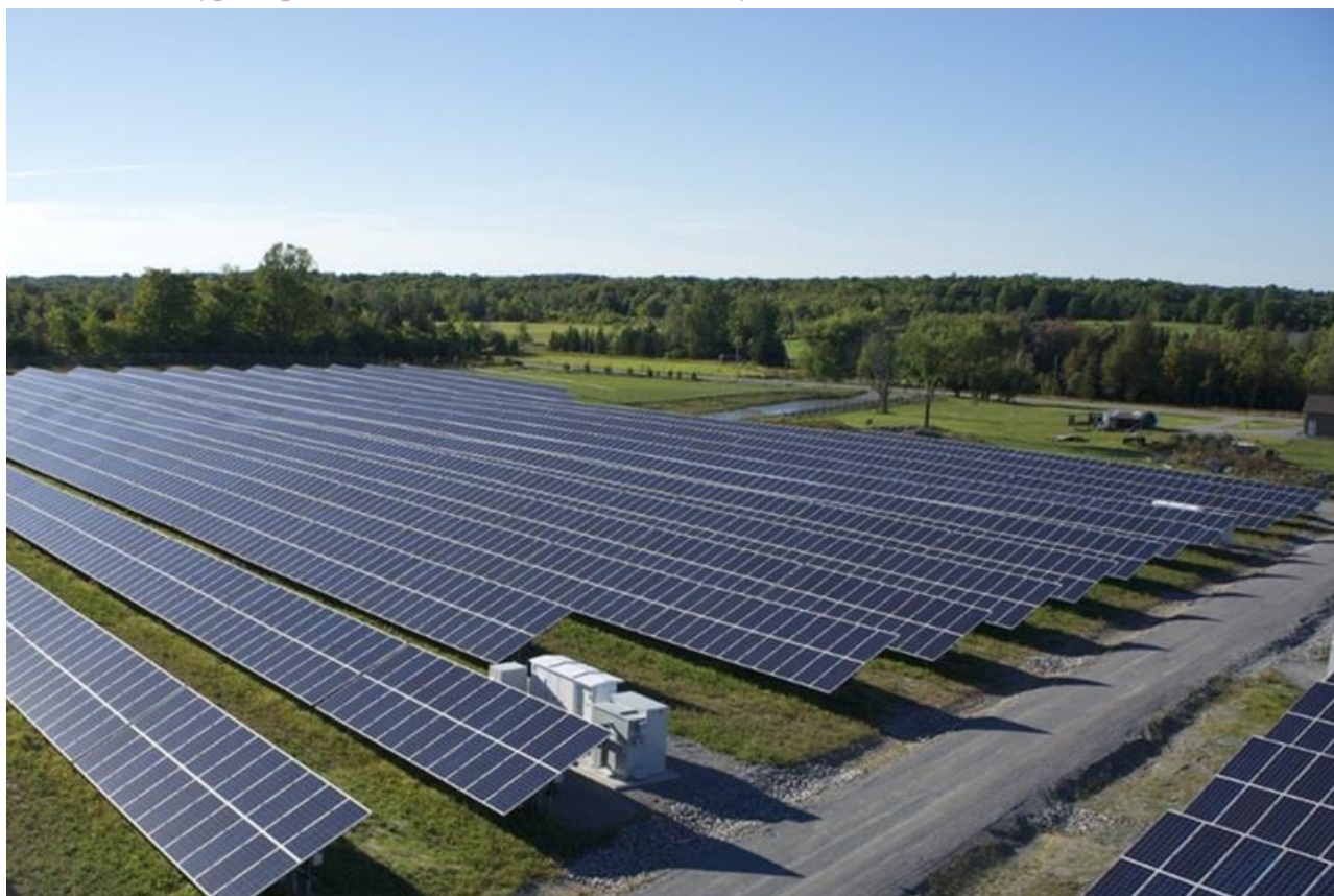
Plate 2-2 Typical photo of tracking solar PV mounted arrays
