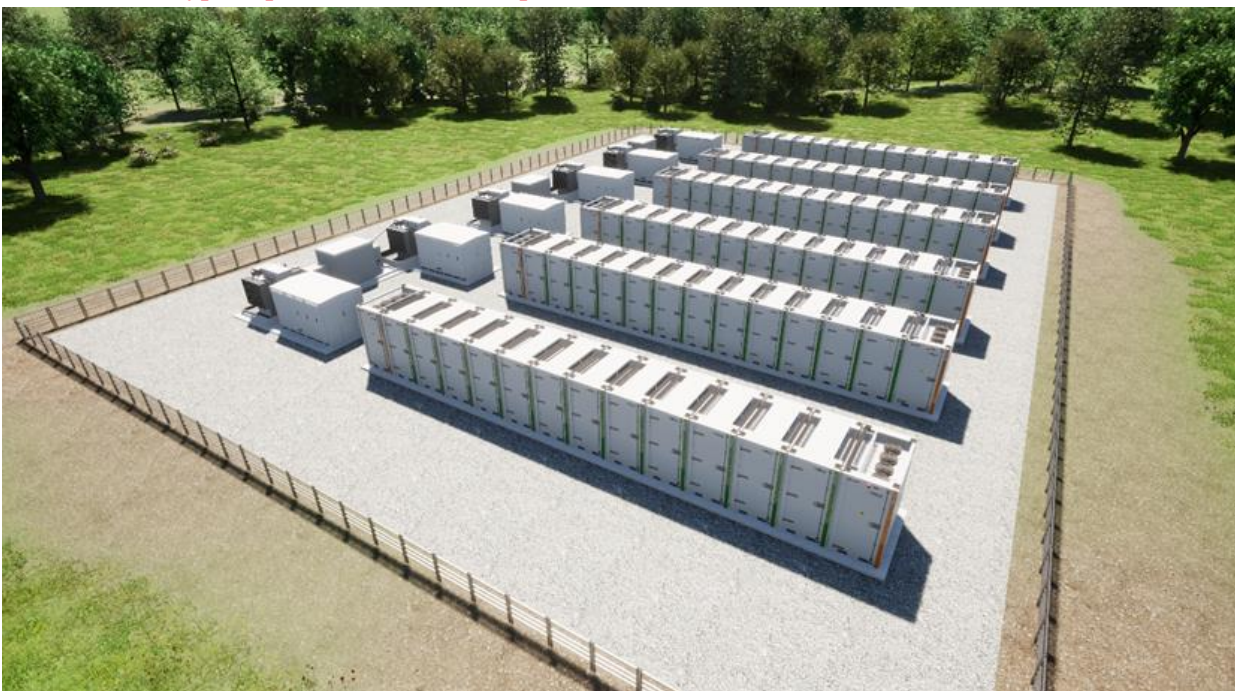
Plate 2-3 Typical photo of a BESS compound
